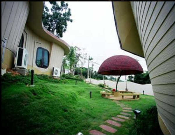
OONRAK SAMUI KENDERGARTEN Samui, Thailand Educational Building Architectural Design Completion year 2005
